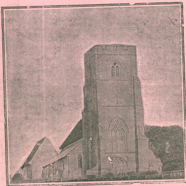
(Tower prior to fall — from an old photograph.)
